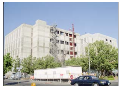
The new Fresno County Jail at Fresno and M Streets nearing completion.
