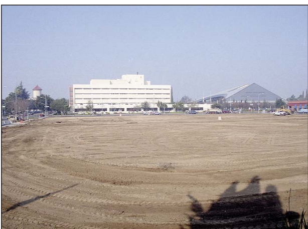
The ground has been cleared for the building of the Robert E. Coyle Federal District Courthouse.
